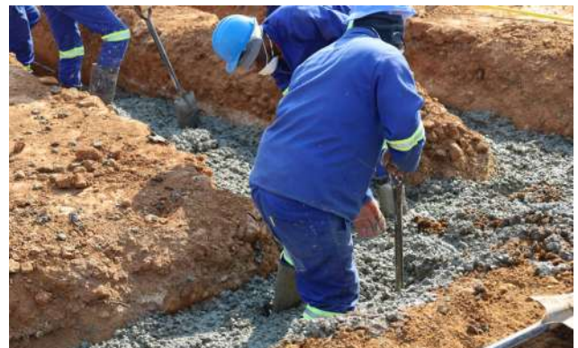
Construction Workers digging the school foundation.
