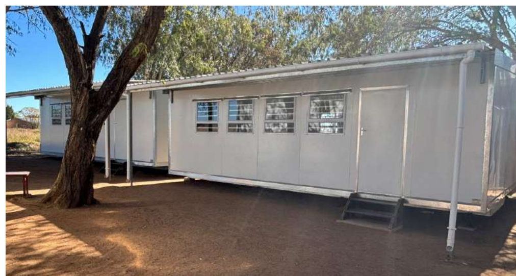
Mobile classrooms provided as a temporary relief to learners of Motlhare Mokautu Secondary School.
