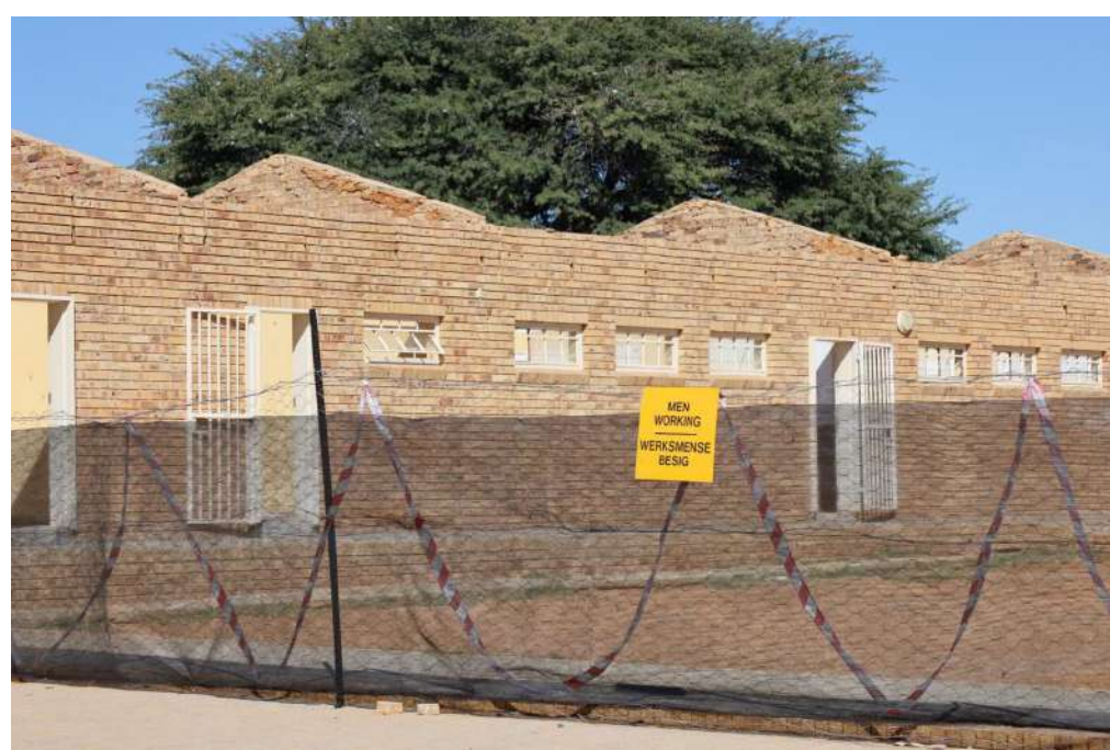
Old Matloding Primary School buildings.
