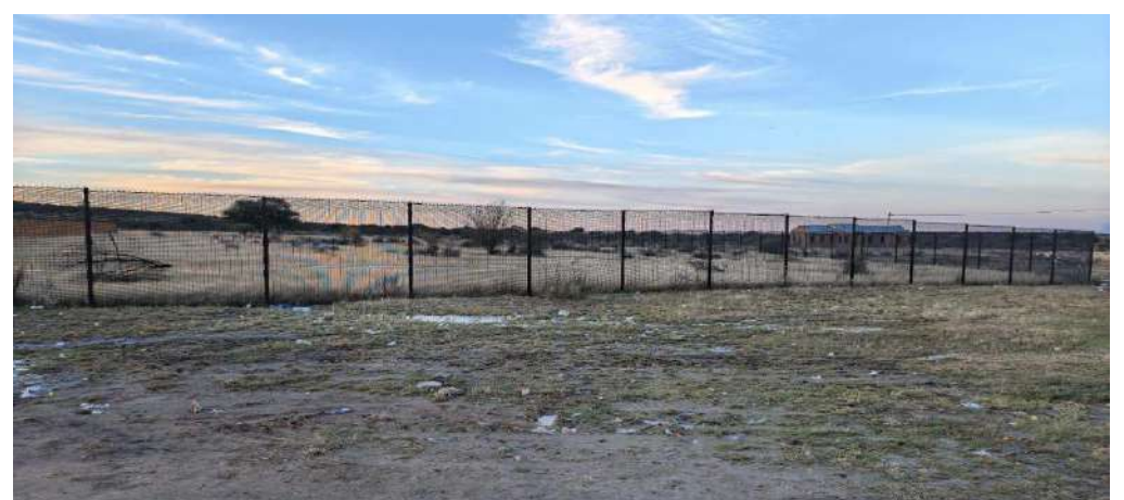
The newly erected fence of Shaleng and Mothelesi Replacement Schools.
