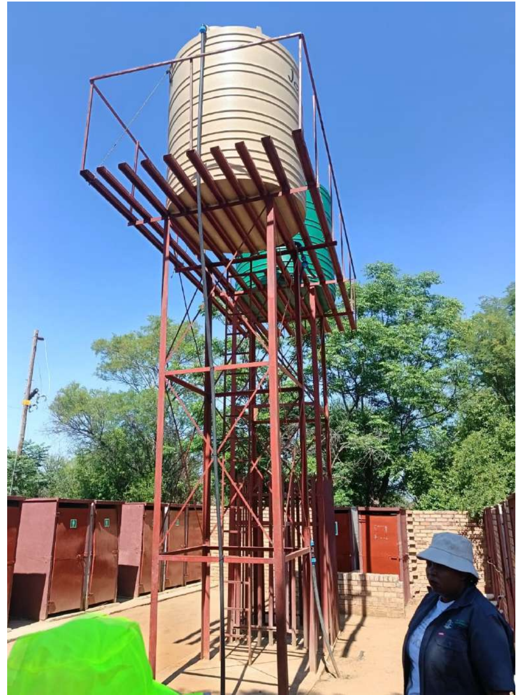
Borehole installed at Molelwane Primary School.
